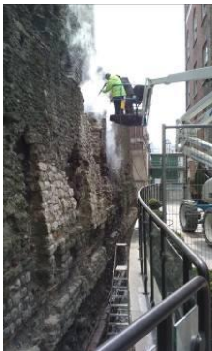
Figure 18 - The author using conservation-grade ThermoTech® equipment on the west elevation
