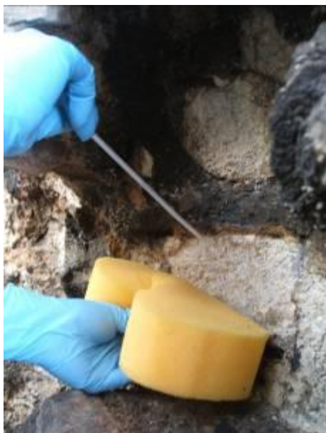
Figure 22 - Applying Calosil E25 by pipette
