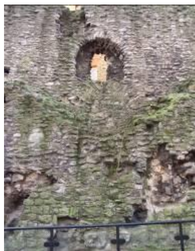
Figure 9 - Zone M3, west elevation
